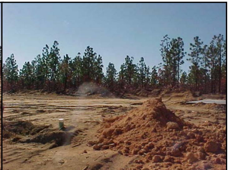
Looking at phase 2 from the site
