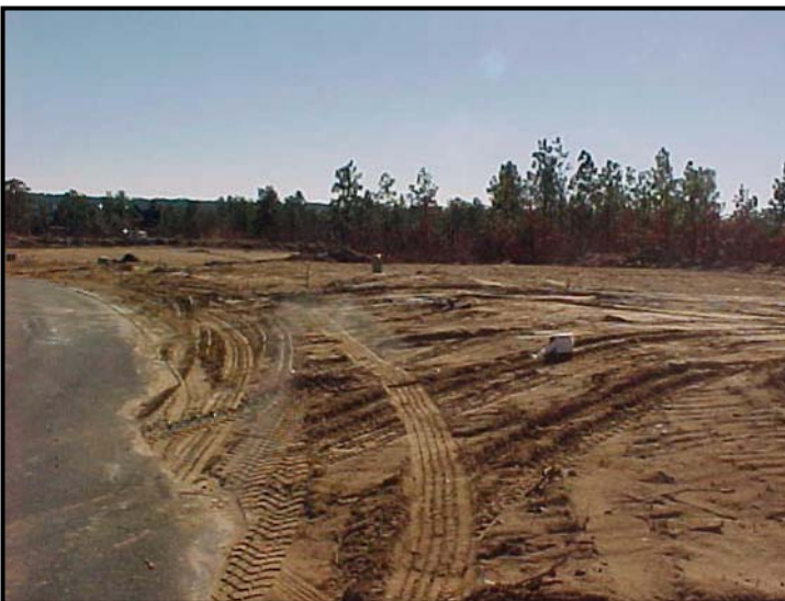
Looking at the site from phase 2
