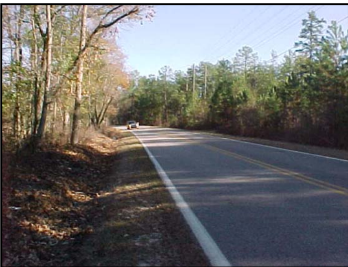
Looking east on Campground Rd.
