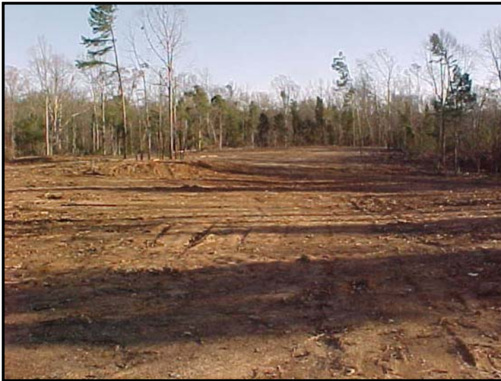
Looking at interior of the site
